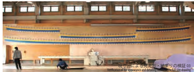
軒廻り現寸図と軒反り曲線 Full-size eaves drawing and eaves camber line
