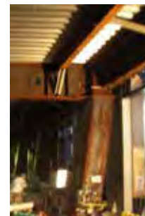
斜柱 (施工中) Slanting columns (under construction)
