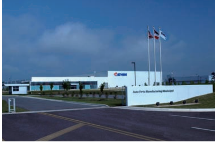
■ APMM New Factory Project ■ U.S.A. ■ Auto Parts Manufacturing Mississippi, Inc.
