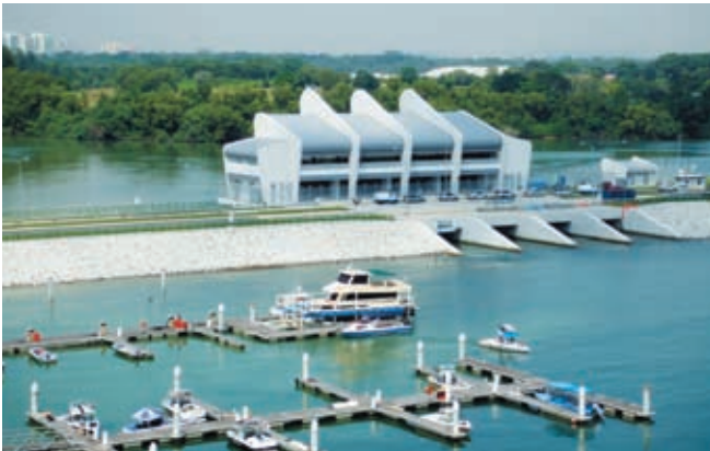
■ Dams, Gates, Dredging and Ancillary Works for Punggol Reservoir ■ Singapore ■ Public Utilities Board
