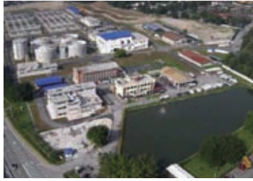
2 Sewage Treatment Plant
