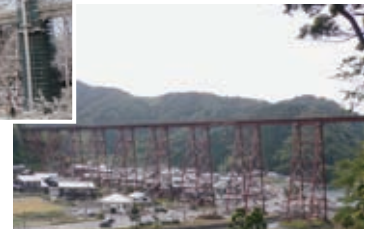
The existing Amarube Viaduct is 41.5 meters high and 309.4 meters long.
