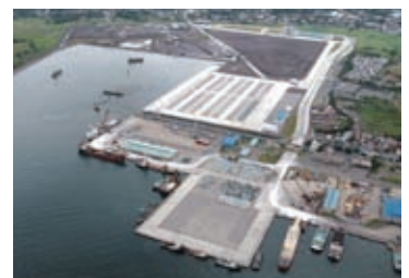
10 Batangas International Container Terminal
