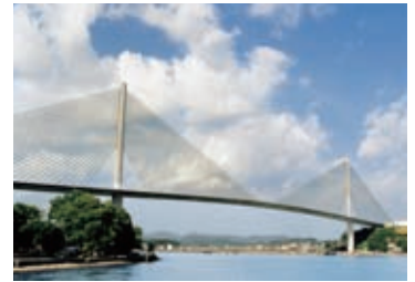
4 Bai Chay Bridge
