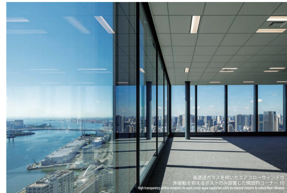
基準階東側内観 柱スパンは18m、天井高は3,000mm 09 East-facing standard floor interior. Featuring an 18-meter column span and a generous ceiling height of 3,000 mm
