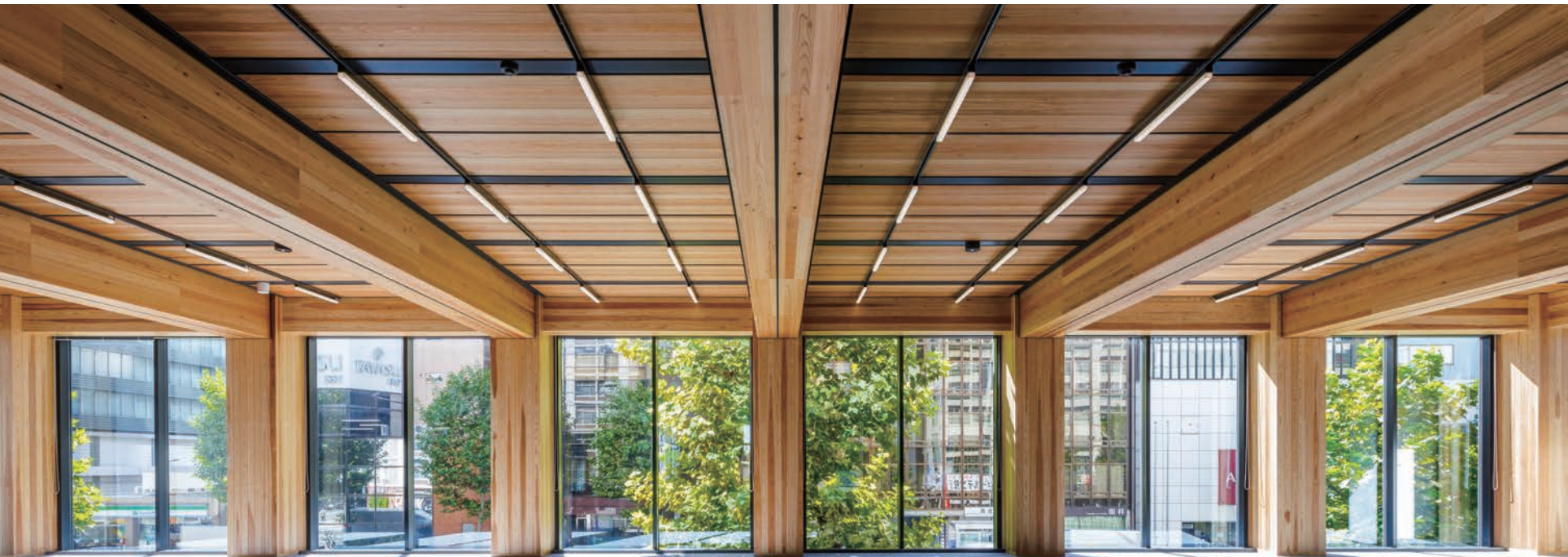
事務室から外堀通りを望む：外周部の柱梁は2h耐火認定を取得した「スリム耐火ウッド®」、天井面の梁は1h耐火となる高層階は「ハイウッドビーム」、2h耐火となる低層階は鉄骨梁の上不燃木練付したO3。View of Sotobori Dori from the office. The outer perimeter columns and beams are made of "Slim Fire-Resistant Wood®", which has obtained a two-hour fire resistance certification. The ceiling beams are made of "Hy-wood Beam" for the upper floors, becoming one-hour fire-resistant, while steel beams finished with noncombustible wood are used for the lower floors, becoming two-hour fire-resistant.
