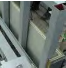
仮置場で組柱に外壁を取付 Outer wall is connected to connected columns in the temporary staging area
