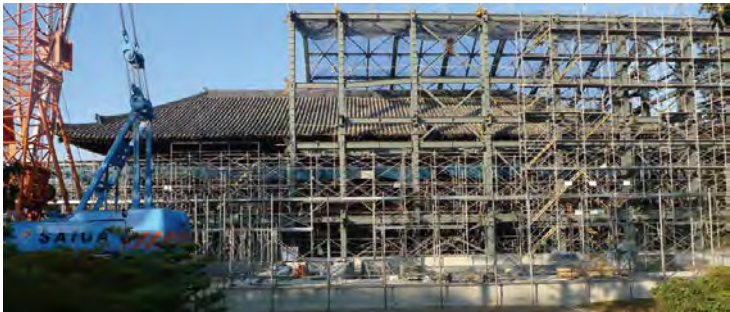
素屋根建方 Erection of covering roof
