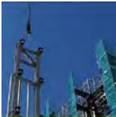
地組された組柱を仮置場に設置 Connected columns assembled at the site are placed in the temporary staging area
