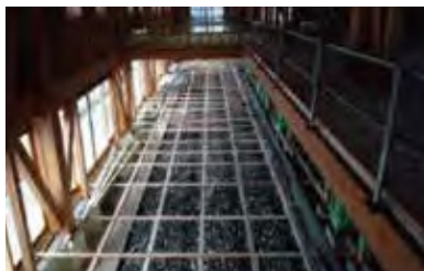
床下蓄熱材 Below-floor heat storage material
