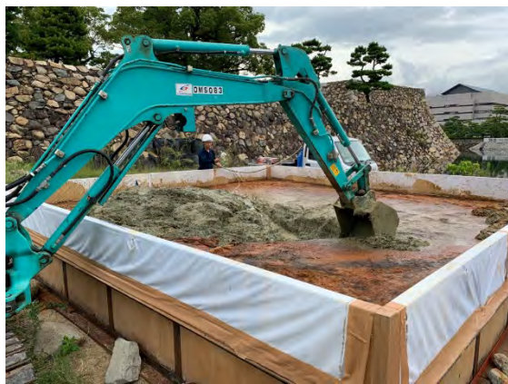
It is being mixed while adding water. The fermentation of straw susa (crack prevention material) has progressed.
