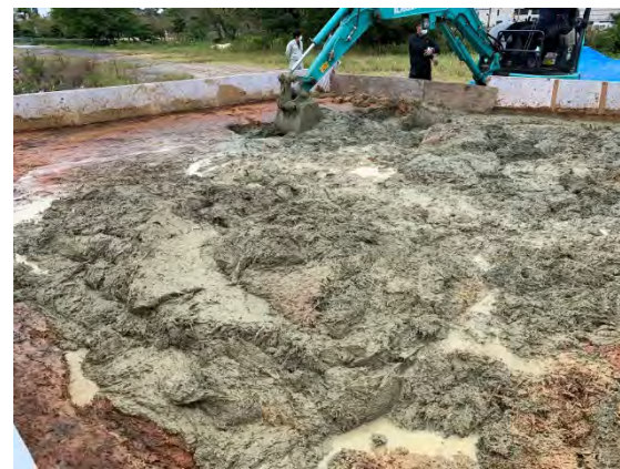
It is being mixed while adding water. The fermentation of straw susa (crack prevention material) has progressed.
