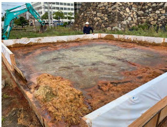
The second mixing of wall clay made at the end of June was done. It is the situation before it.
