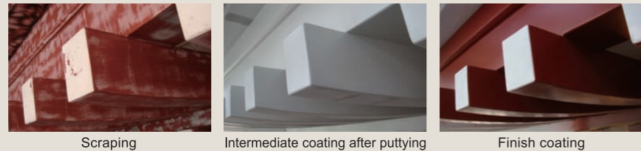
Scraping Intermediate coating after puttying Finish coating
