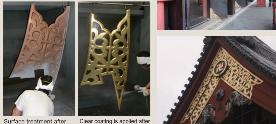
Surface treatment after removal Clear coating is applied after impressing gold foils on it
