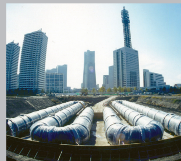
災害用地下給水タンク (50万人分の飲料水3日分供給可能) Emergency underground water tank (Storage of a three-day supply of drinking water for a half million people)
