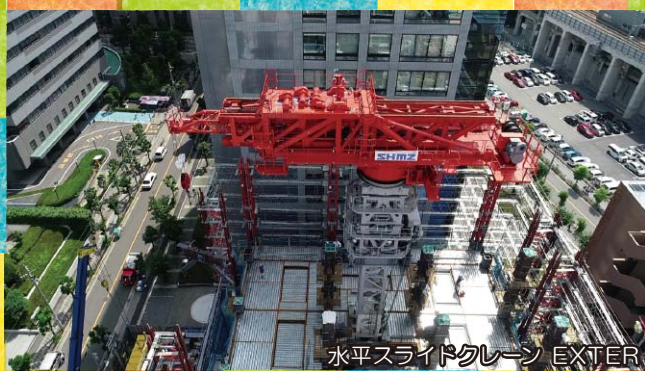
Shimz Smart Site
