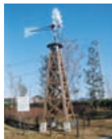
Wind-driven groundwater pumping system
