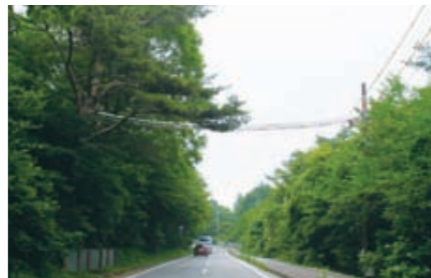
An animal pathway installed over a road in Hokuto City
