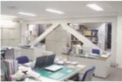
An office reinforced with seismic braces and other devices. Safety has been improved significantly to ensure that the building can continue to be used with peace of mind.
