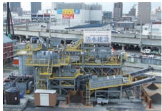
On-site soil washing plant dealing with small-scale projects that started operation in May 2008
