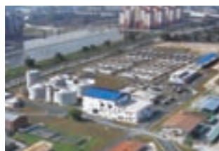
The sewage treatment plant in Malaysia near completion. The pond on the far left is the treatment plant currently used.
