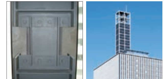
(left) Steel stud damper*2. Both steel stud dampers and oil dampers*1 are maintenance-free and exchangeable. (right) Approximately 50-meter-tall steel telecommunication tower
