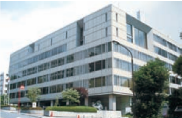
Kikai Shinko Kaikan building
