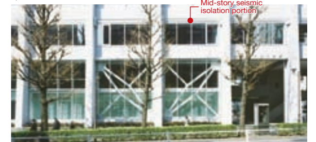
The change in the external appearance of the mid-story seismic isolation portion was minimized. For the floors below the seismic isolation layer, vibration control was enhanced by installing neat-looking toggle dampers.*3
