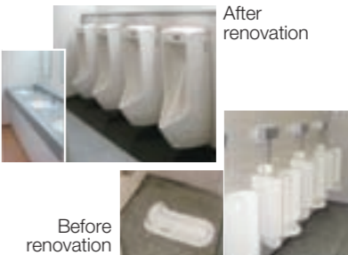
Renewed toilets. In addition to improving amenities for office workers, the new toilets—equipped with the latest water-saving technology—are also effective in decreasing both water use and sewage disposal, thus minimizing their environmental impact.
