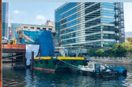
A temporary pier enabled transportation of excavated soil away from site by boat
