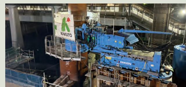
Gyropress use in revetment reconstruction
