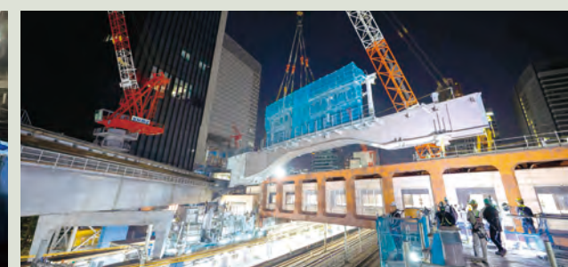
Walkway girder installation above the rail lines
