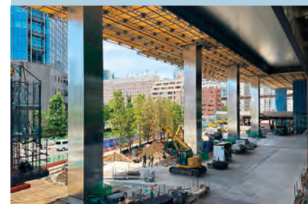
View of the 18-meter span external columns on the first floor
