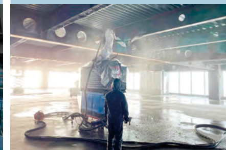
Experimental use of our fire-resistant coating robot
