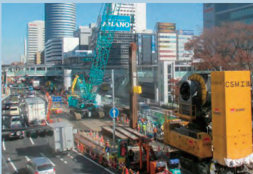
Steel-reinforced continuous underground wall components installed along Circular Line 2
