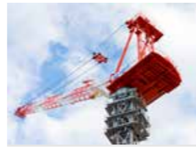
A tower crane, the main work horse
