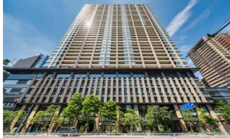
Park Court Bunkyo Koishikawa the Tower (Bunkyo-ku, Tokyo)
