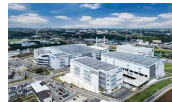
Panoramic view of S.LOGi NIIZA with East 2 in the foreground (Niiza City, Saitama Prefecture)
