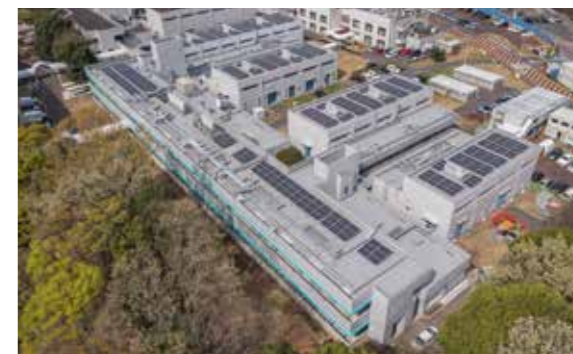
AIST Global Zero Emission Research Center, which achieved ZEB certification through renovation work (Tsukuba, Ibaraki Prefecture)
