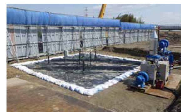
Thermal desorption soil remediation(test facility) (Kuwana City, Mie Prefecture)
