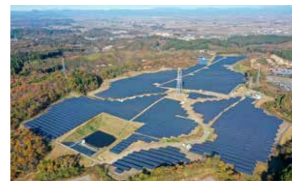
JPS 20 Osaki City Sanbongi Solar Power Plant (11.88 MW generation capacity) (Osaki City, Miyagi Prefecture)
