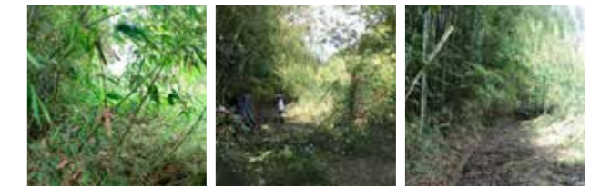
Renewing green infrastructure in uncultivated rice fields Before installation of a water canal (left), during construction (center), restored water canal (right)
