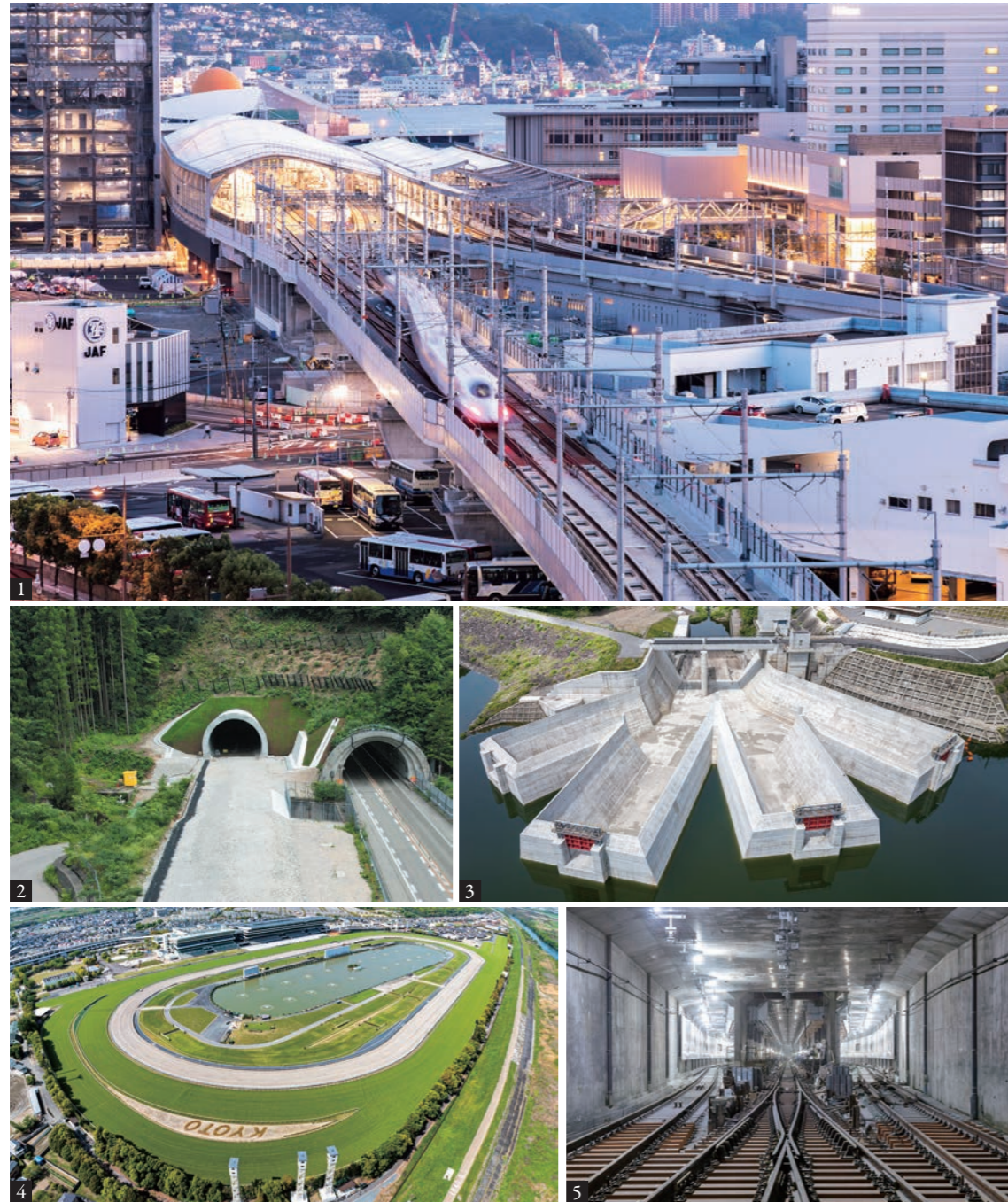
1 The Kyushu Line (West Kyushu), Nagasaki Station Elevated Bridge (Nagasaki, 2023)
