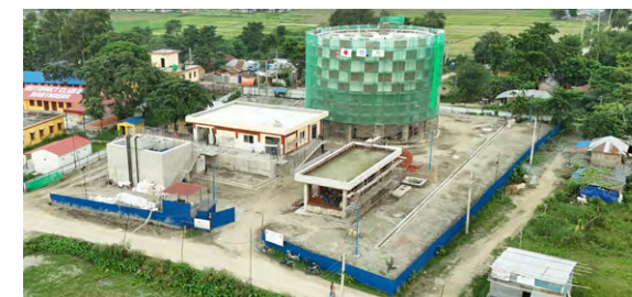
Biratnagar water supply improvement project (Nepal)
