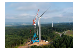
Bird's eye view of the SMTC construction work in action
