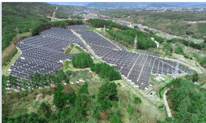
Repowering of the Existing Power Generation Facilities at the Nagano Prefecture Suwa Fujimi MS Solar Power Plant (Suwa City, Nagano Prefecture)
