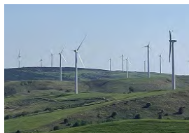
Eurus Soya Misaki Wind Farm (Wakkanai City, Hokkaido)
