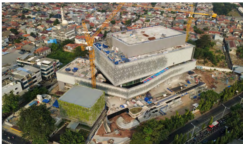
The exterior is largely complete, and finishing work is underway
