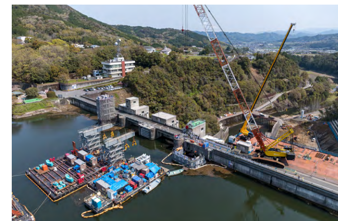
Nomura Dam Facility Improvement Project: Construction using a floating upstream temporary bulkhead (Seiyo City, Ehime Prefecture)
