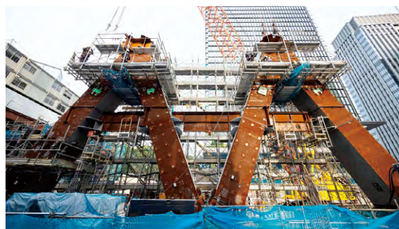
Torch Tower under construction: Diagrid structure (Chiyoda Ward, Tokyo) as of August 2025
