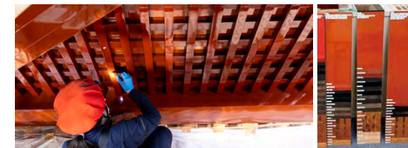
Lacquering with kushimagiri bengara . The lacquering of the building exterior involved as many as 27 processes in some cases.
