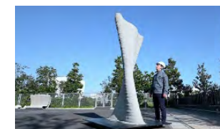
A twisted wall created using a Spray-based 3D concrete printing system
