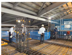
Reinforcement inspection training using mockups
