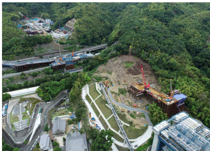
Kajiwarra Tunnel Construction Project Construction is underway on the Shin-Meishin Expressway, Japan's new major artery (Takatsuki City, Osaka Prefecture)
