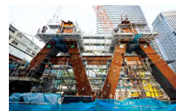
Building Construction ▶ P.35
