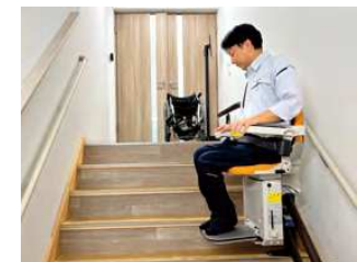
Construction site office lift for wheelchair users
