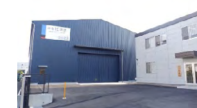
Exterior view of TAKUMI TRAINING CENTER (Funabashi-shi, Chiba Prefecture)
