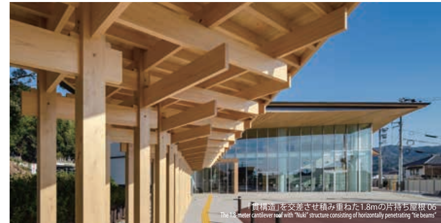
県産木材の流通製材による木造のキャノピー 05 Wooden canopy made of commercially available lumber based on prefectural wood
