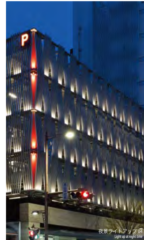
北国パークビル 03 Overall view on north-west side
