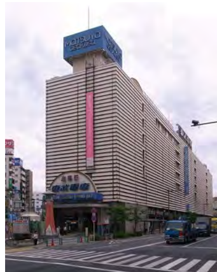
改修前 Before renovation
