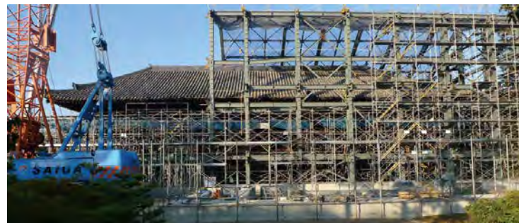
素屋根建方 Erection of covering roof
