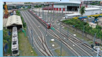
Philippines LRT 1 line vehicle depot
