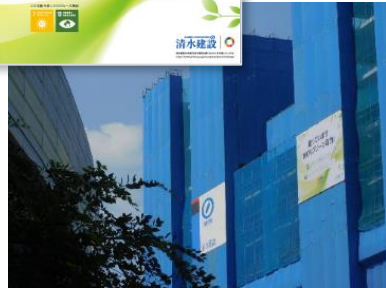
PR with temporary enclosed signboard, mesh sheet
