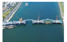
(3) Second arch construction (afternoon of May 17)
