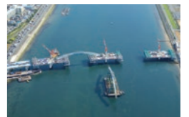
(2) Second arch towing (morning of May 17)
