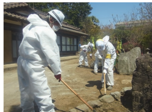
Decontaminating a home (in the Tomioka decontamination project currently underway)
