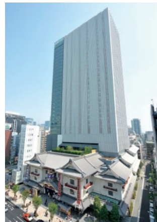
Ginza Kabukiza (construction) Photo courtesy Shochiku Co., Ltd. and Kabuki Za Co., Ltd. (Photo taken May 2013)
