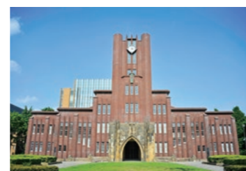
Yasuda Auditorium after repairs
