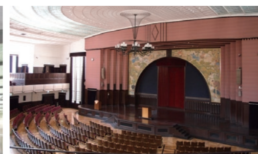
Inside the auditorium after repairs
