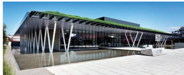
Yanmar Museum (construction)
