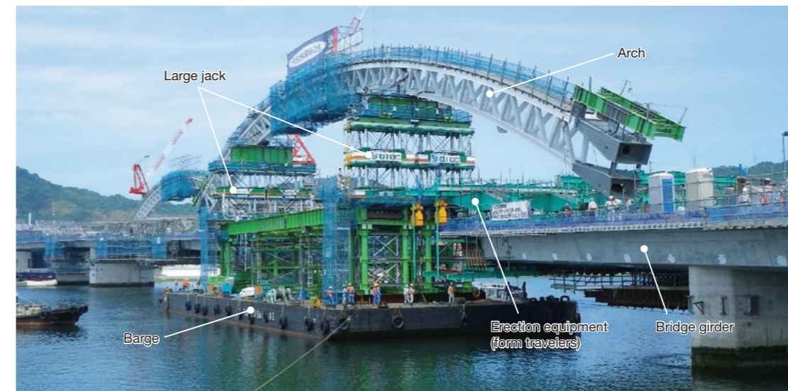
condition of second arch construction (May 17 in 2013)
