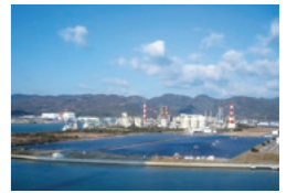
A solar power project (Ako Solar Power Company)
