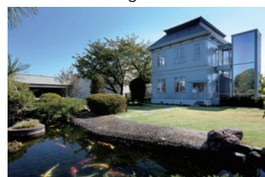
Seifun Museum, main building (repairs design/repairs construction)
