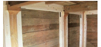
Reinforcing beams and pillars (lighter-colored material is reinforcement)
