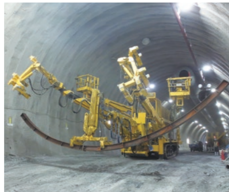
Invert strut installation robot
