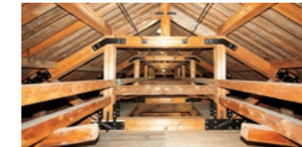
Repairing and improving the truss
