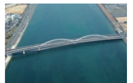
(5) The completed Otagawa Ohashi Bridge
