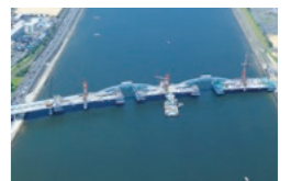
(4) Balanced cantilever erection (block 9 and later)
