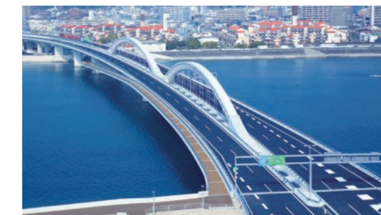
The completed Otagawa Ohashi Bridge
