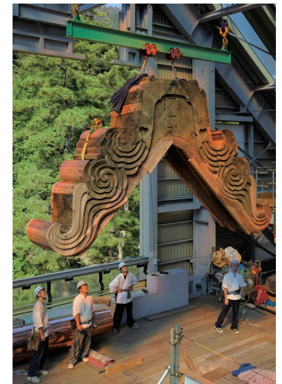
A Installing a restored ridge-end ornament
