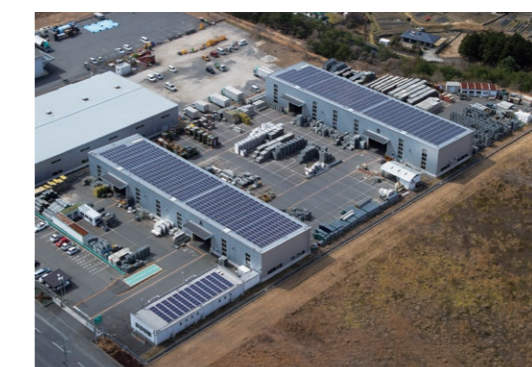
Solar power facilities at the Hiroshima Materials Center
