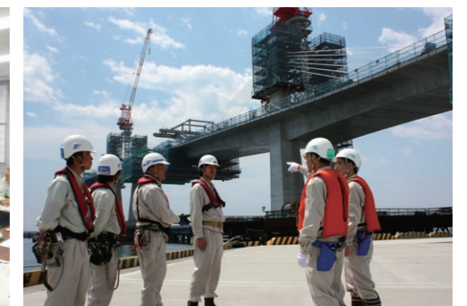
A site patrol during concrete work
