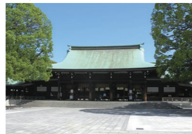
Meiji Jingu Gehaiden (construction for earthquake proofing reinforcement)
