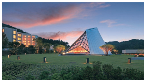
Chapel, Miho Institute of Aesthetics (construction)
