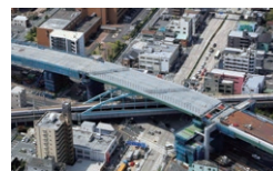
⑤ Rotating the bridge girders and connecting them to girders on each side
