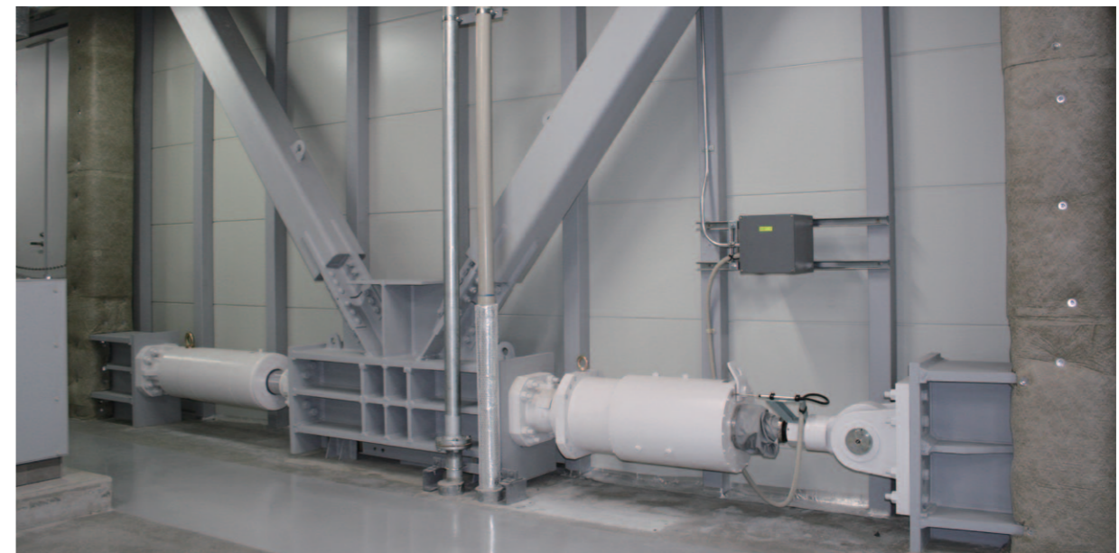
Example of Dynamic Screw damper installation
