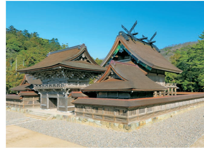
A The completed main shrine
