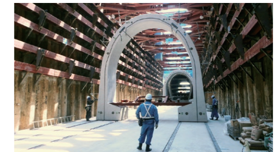
The tunnel restored with Modularch members
