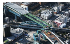
② After first launch (the tip of the launching girder has reached its destination)
