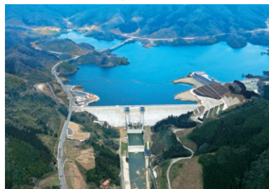
Construction of Obara Dam
