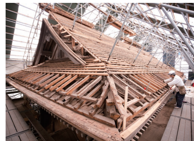
B Restoration of a structure known as "Kansairo"
