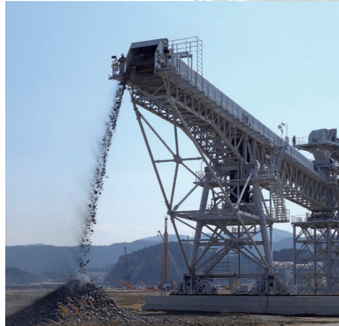
The massive conveyor belt used to transport earth
