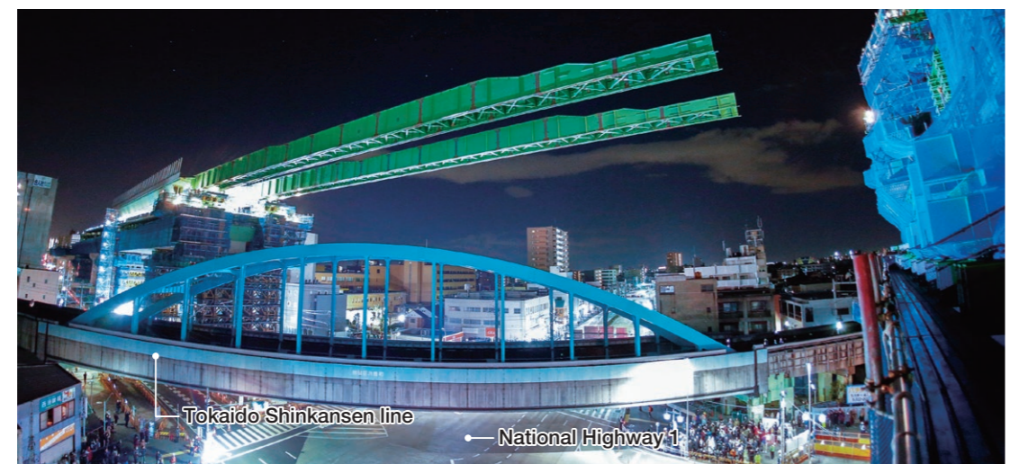
Launching bridge girder
