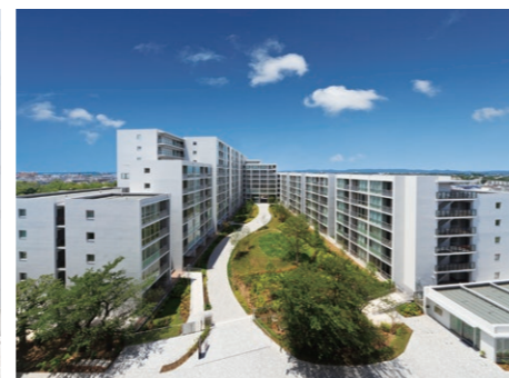
Gardenier Kinuta West, eco-friendly, disaster-resistant condominium project by Shimizu design and build
