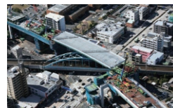
④ After 11 launches (Completion of launching)
