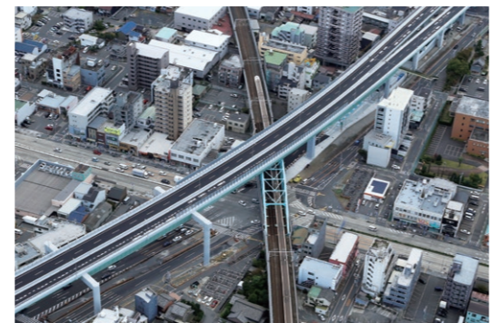
The completed Rokubancho Overpass
