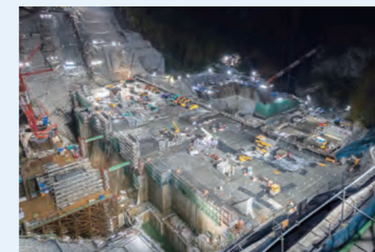
Construction work using ICT in progress on Yamba Dam
