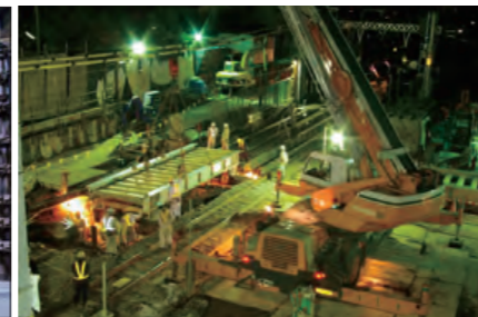
Japan's first grade separation project to increase the number of lines to a 4-line subway directly beneath an operating railway line — Completion of Rail Rapid Transit (RRT) Line No. 9 — Odakyu Electric Railway Co., Ltd. Odawara Line
