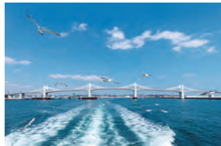
Onahama Marine Bridge
