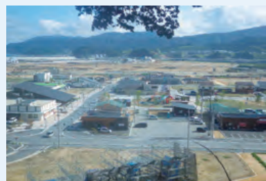
Progress on home construction on the delivered development in the Takata district of Rikuzentakata City
