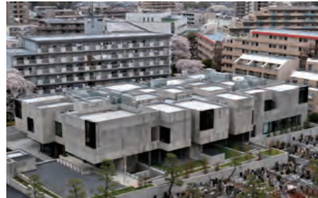
Building No. 1, Toho Gakuen College Chofu Campus (building construction)
