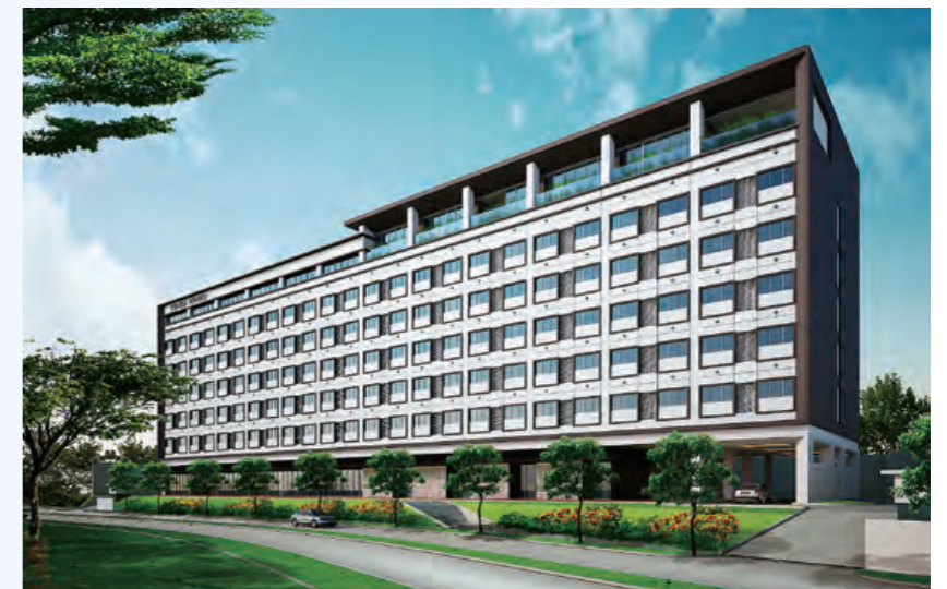
The Cikarang serviced apartment project under development in an industrial park on the eastern side of Jakarta.
