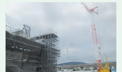
A latest crawler crane
