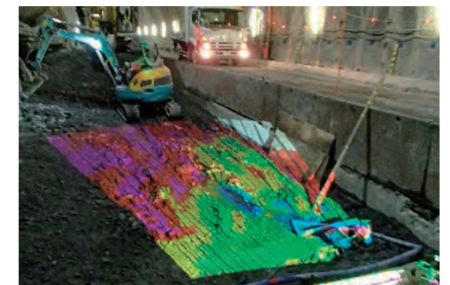
Imaging data projected on the floor of an invert
