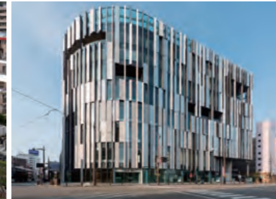
Toyama Glass Art Museum (building construction)
